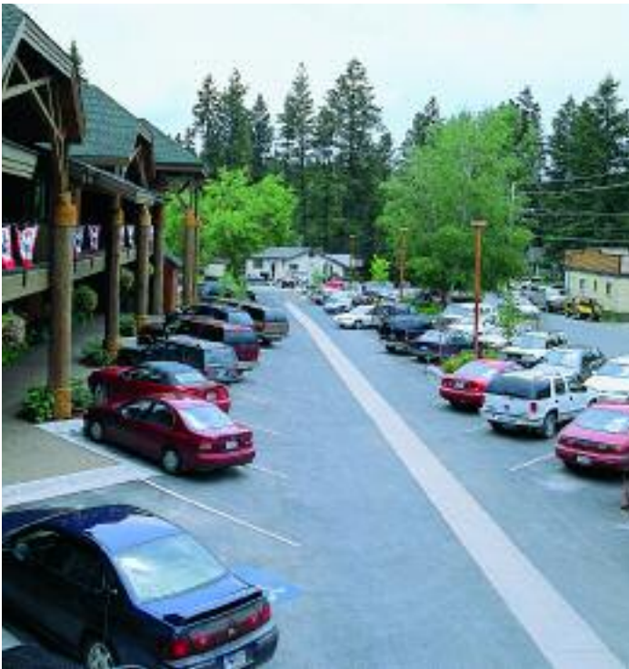
On the cover: Rainstore³ chamber under parking lot, Broomfield, CO. Without Rainstore³'s high water storage capacity at shallow depths, the flexibility in design, and the convenience of exfiltration, the owners of this site would have been unable to develop this site and would have been forced to find a different location for their new construction.
