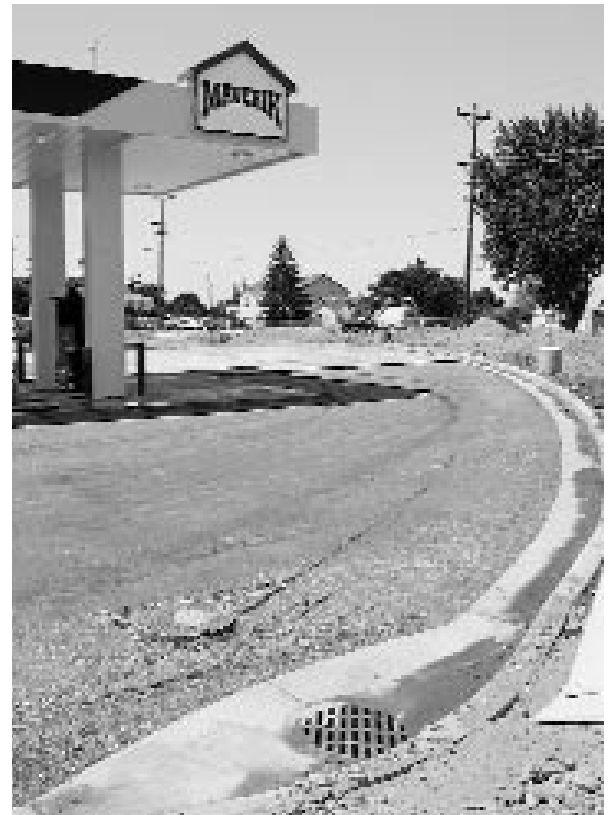
Above: Nearly completed installation of a stormwater detention system at a gas station in Nampa, ID. This site has three separate Rainstore 3 chambers to provide the necessary water storage. This photo shows the catch basin and curbing for one of the chambers. Asphalt will cover the visible gravel base.
