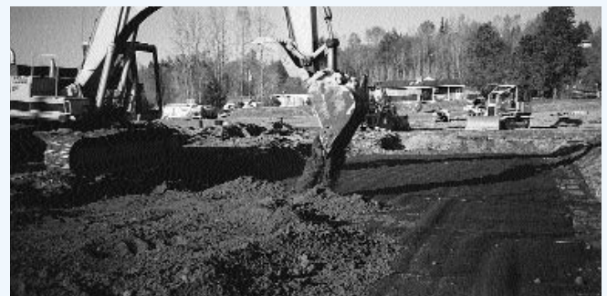
Backfill with roadbase prior to operating heavy machinery on Rainstore 3 units
