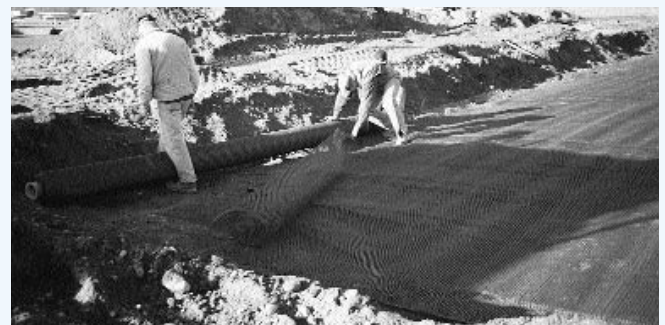
Filter fabric with geogrid placed on top
