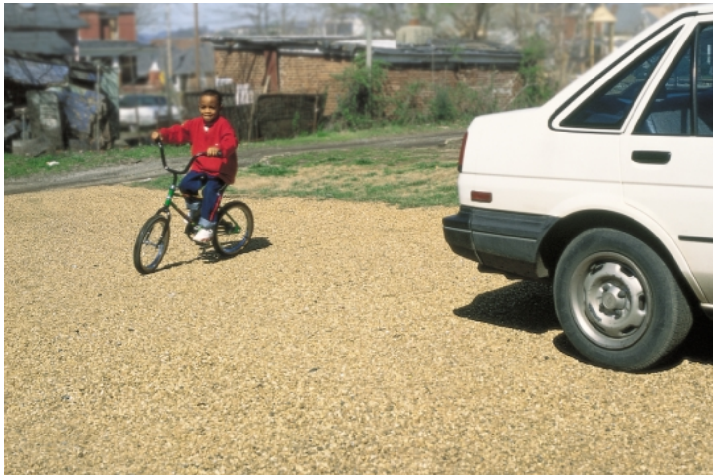
Fort Negley, Chattanooga Neighborhood Enterprise, Chattanooga, TN — Driveway is stable for auto, bicycle and pedestrian traffic on this two-year-old surface, while allowing storm water infiltration. Note the absence of weeds and car oil stains.
