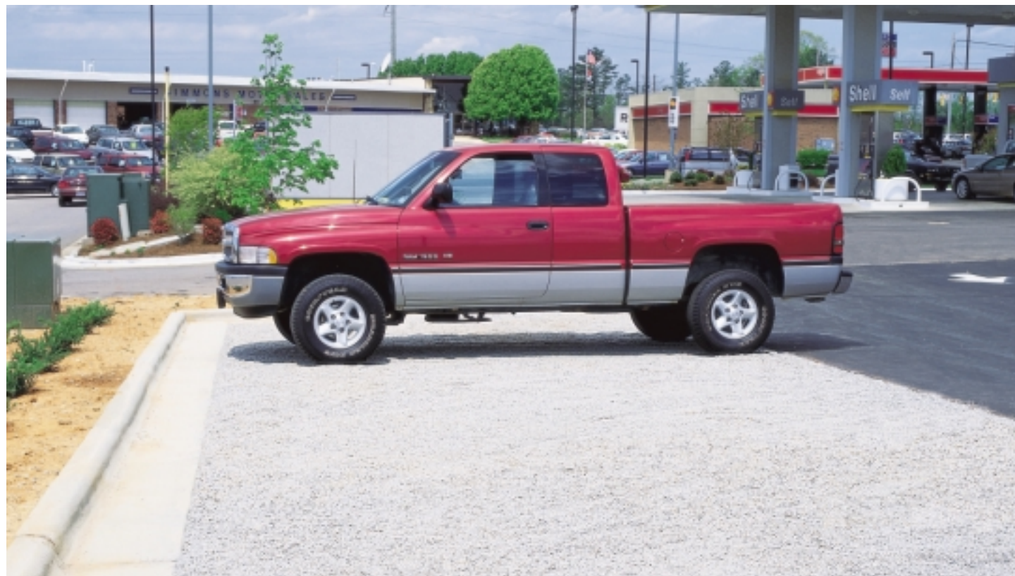
Taco Bell, Henderson, NC — Remote gravel parking bays receive storm water from asphalt areas.
