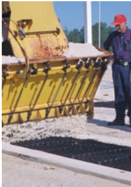
Stone chipper machine distributing gravel fill at University of South Alabama, Mobile, AL.
