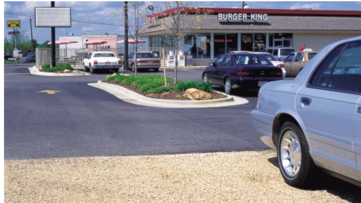
Burger King, Henderson, NC — Porous parking areas around building. Asphalt areas are graded to drain into the Gravelpave 2 bays.
