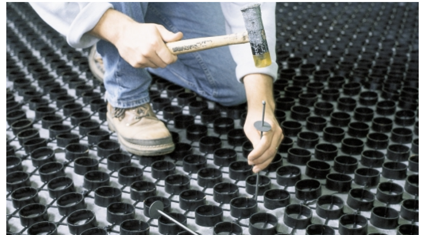
Anchor pins are used to secure rolls to base course.
