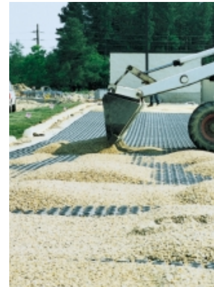
Front-end loader distributes gravel fill at Burger King, Henderson, NC.
