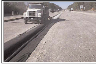
Trench was wrapped with Mirafi 140NC, fitted with 6" ADS pipe and backfilled with stone
